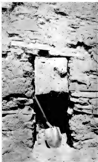
Doorway connecting interior rooms at Pueblo San Cristóbal. This is the form of door in general use in all the pueblos of the region
